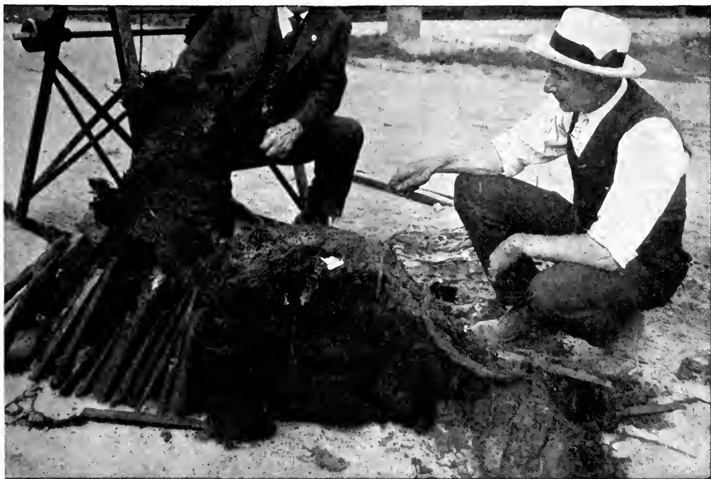
A MASS OF LARGE ROOTS TAKEN FROM A 24-INCH SEWER AT ANTIGO, WIS.
